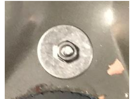
Installed Bolt with Fender and Lock Washer
